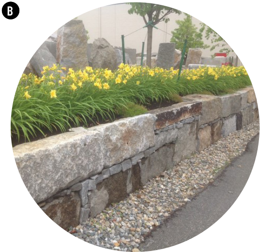
QUARRY BLOCK RETAINING WALL/BENCH
