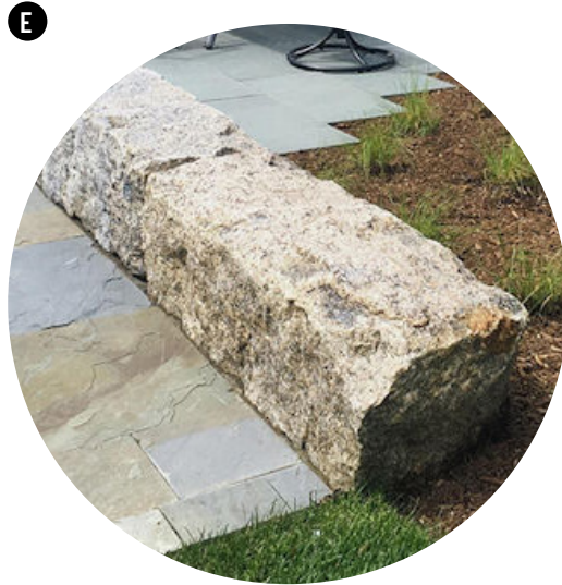
QUARRY BLOCK RETAINING WALL/BENCH
