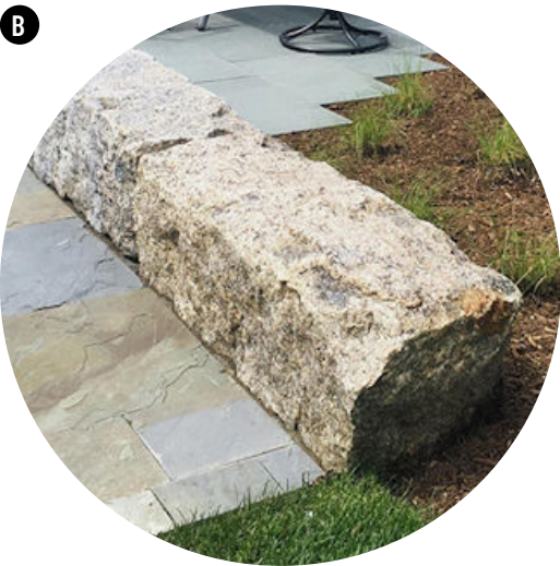
QUARRY BLOCK RETAINING WALL/BENCH
