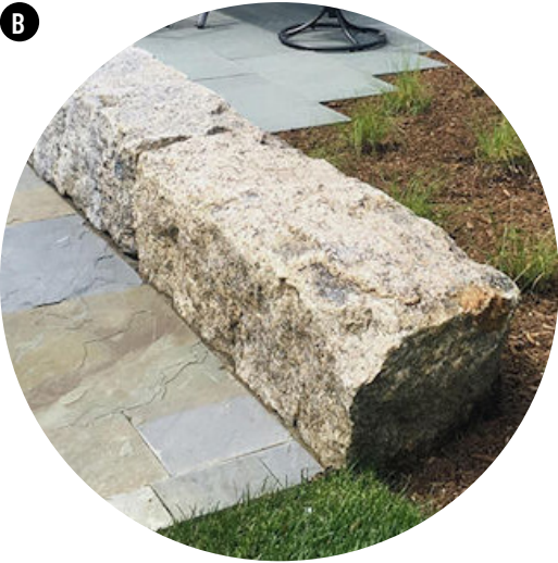
QUARRY BLOCK RETAINING WALL/BENCH
